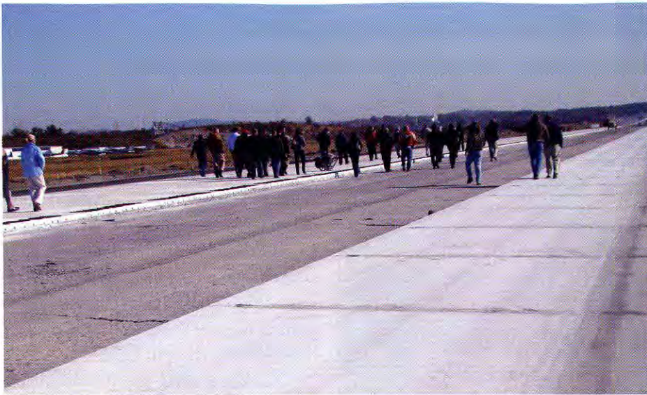
Pavement was placed in 25-foot-wide strips—with subsequent infilling between.
