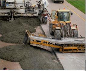
The conveyor is conveniently controlled from the loader controls inside the cab of the loader. The speed of the belt is controlled by the engine RPM and the flow of oil through the control values. The folding and travel features are controlled from auxiliary controls on the conveyor base at ground level.
