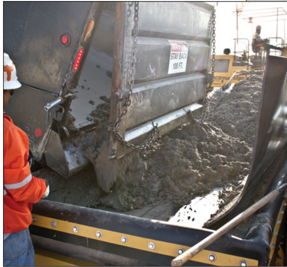
The Portable Modular Conveyor-Material Placer at work on a Tulsa Airport project.
