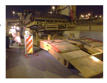
hopper was plenty large enough to handle large loads, the extra capacity was not needed for this project, because the conveyor moved the ballast into place within seconds.
